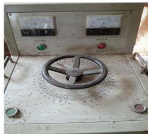
(a) Current generator
