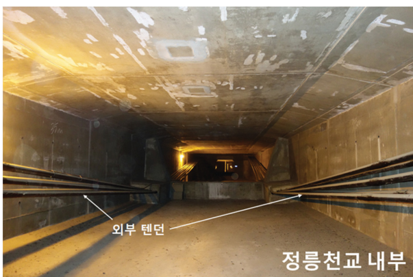
Fig. 1. (Color online) Internal of box girder in Jeongrung bridge.
